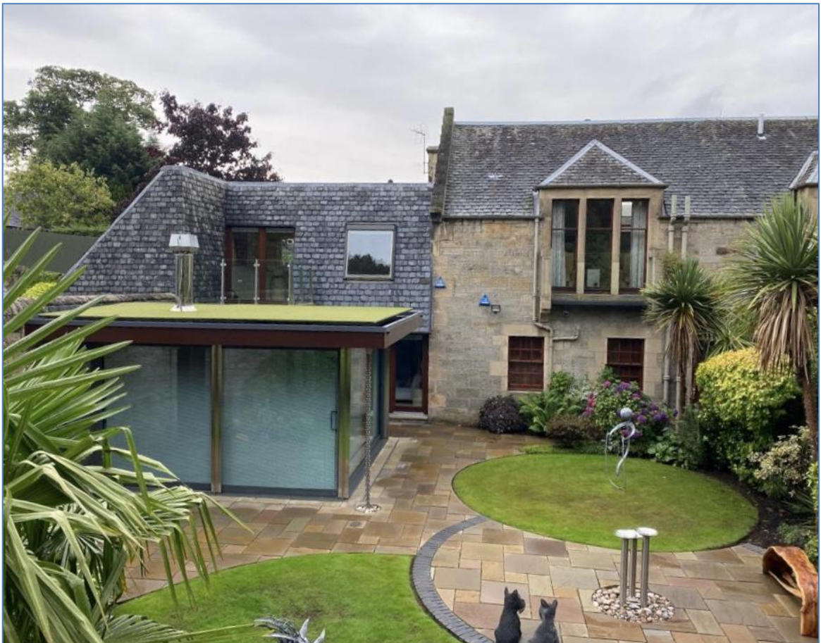
Figure 11: 35 Ravelston Dykes Road rear glazed modern extension. This property used to form a larger property with No. 39 (the appeal site) - see also Figure 5 which shows both No. 35 and 39 alongside each other.
