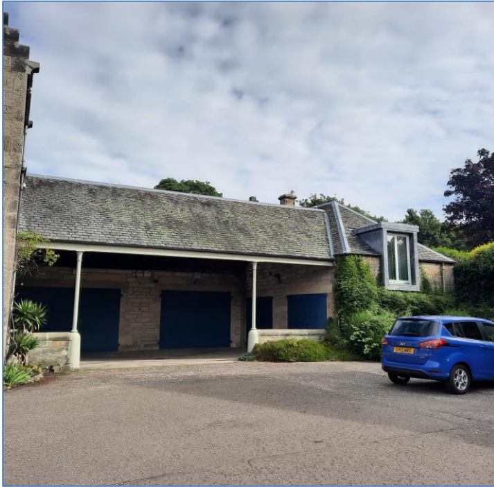
Figures 12 and 13: the former shows a new vertical window in No. 35 Ravelston Dykes Road in full public view. The latter shows a modern extension at No. 37 Ravelston Dykes Road. A consistent approach should be applied at No. 39 Ravelston Dykes Road.
