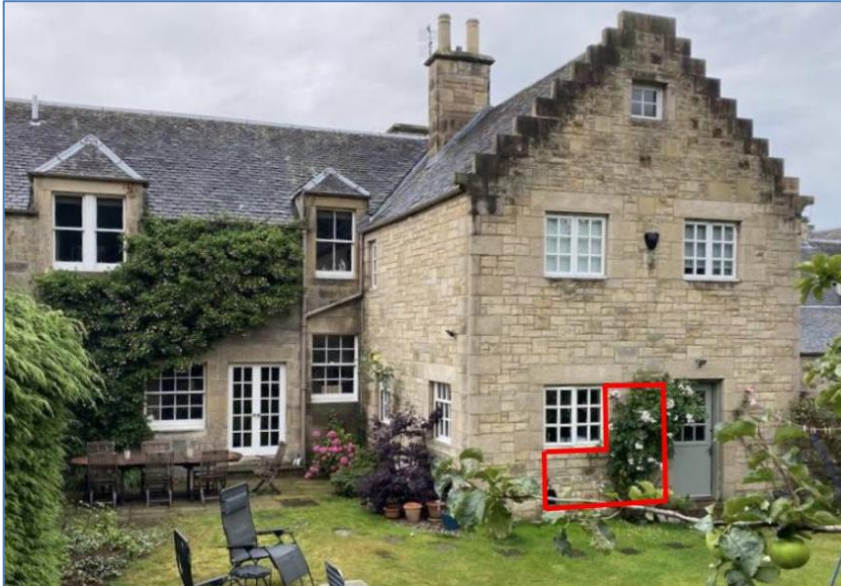
Figure 4: The red line shows the extent of the new glazed opening to be created on the pastiche modern 2000 extension
